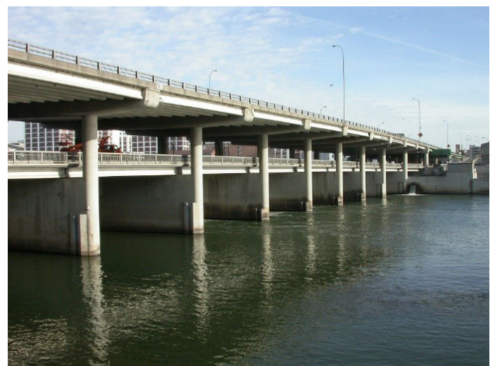
5 in 1 Bridge carrying I-380 and city streets over the Cedar River dam
